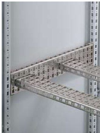
Grid strap installation (from side to side).
