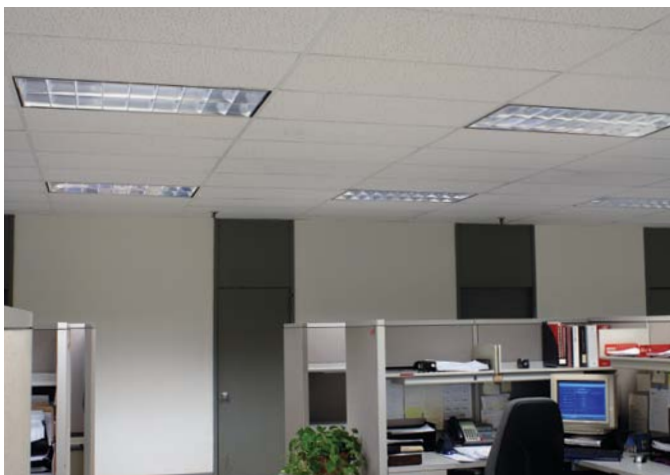
The sharp cut-off of a traditional parabolic fixture casts dark shadows on the wall creating a cave effect.
