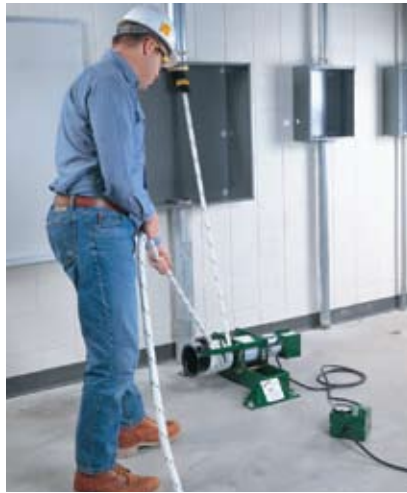
Operator is making a downward pull from the box using the puller with the floor mount anchored to the floor.
