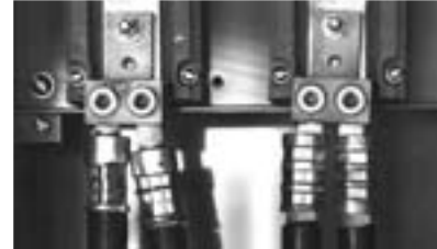
Lug Will Not Accept Straight Pin Offset Pin Design - Application
