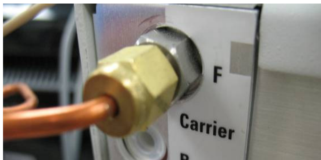
Figure 488. Plumbing the Nitrogen Supply to the GC
