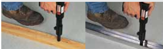
2" x 4" to concrete slab
