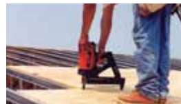
Plywood attachment—using TrakFast plywood to steel pin
