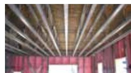
OSB and plywood to iSPAN joists
