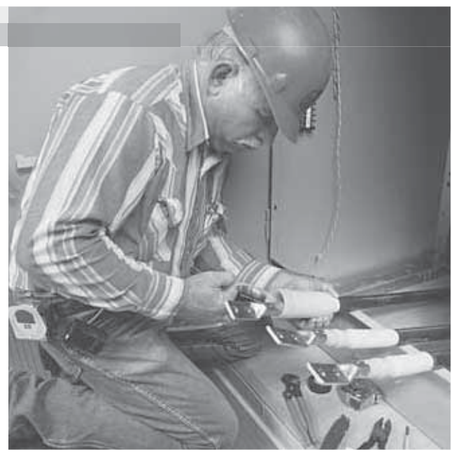
3M™ Cold Shrink QT-II Indoor Termination
