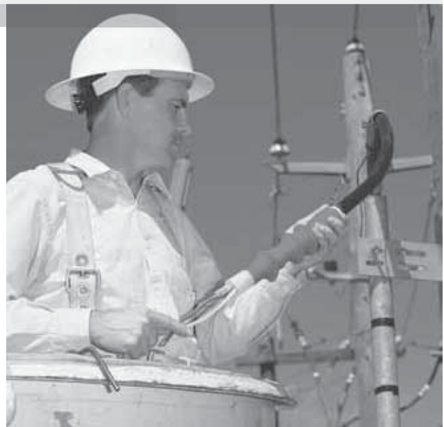
3M™ Cold Shrink QT-III Outdoor Termination
