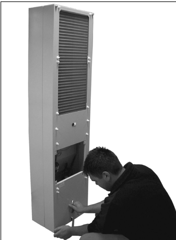
Fig. 74: Loosen the four nuts of the cover
