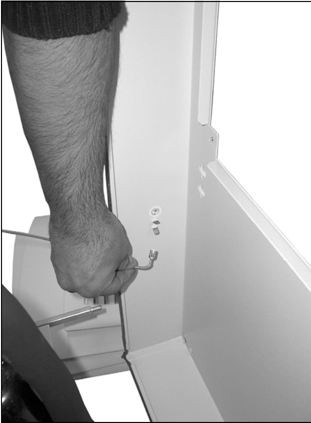
Fig. 77: Disconnect the earthing cable (2)
