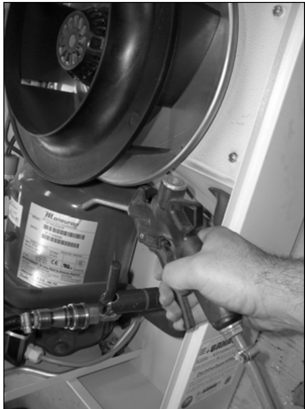
Fig. 80: Clean out the heat exchanger coil and compressor chamber using compressed air (3)
