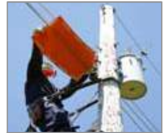
Installing a Zip-On Blanket
