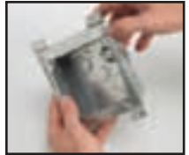
4. With the tabs closed, the box remains secured to the bracket when the plaster ring is removed
