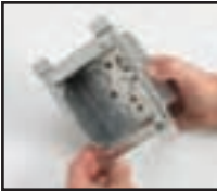
2. Insert box screws into open slots
