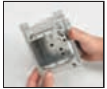
3. When plaster ring is installed, the ear tabs are bent down into the closed position
