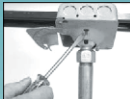
Rotate fixture so slot in pivot aligns with T-tab in cover. Press the T-tab into the pivot.
