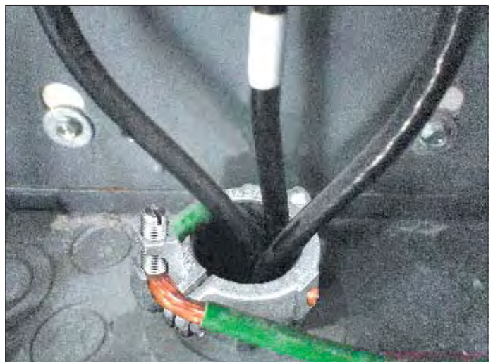
SPLIT-COLLAR GROUNDING BUSHING
