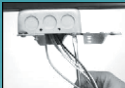
Mount cover plate (with its door open) onto the ceiling box.
