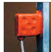
FSPD APPLIED TO ELECTRICAL BOX
