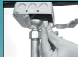
Lift light fixture and set its pivot in place on swivel cover. Connect and dress the wiring.
