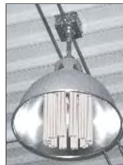
Pan Deck Box Mounting with Hands-Free Hanger
