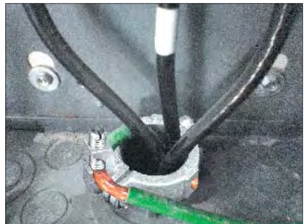
SPLIT-COLLAR GROUNDING BUSHING
