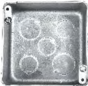
OLD BOX WITH EAR CONVERTERS ADDED
