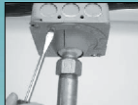
Close the cover door and secure it with screw.
