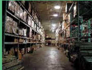
400W Metal Halide Lamps $1000 Annual Energy Cost Operating Temp: 1385°F Costly Heat Load on A/C
