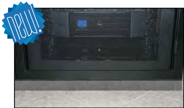
FOAM BLOCKS TO PREVENT BYPASS AIR Please call 1.866.TRY.GLCC for details
