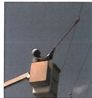
LIVs and LVTs are used throughout the world for overhead conductor voltage isolation verification. 60, 50, or 25 Hz versions are available as standard units
