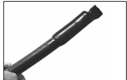
3. HSIC-FR end cap installed on cable.
