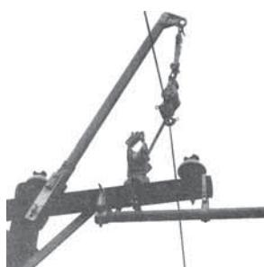
Aluminum alloy base assembly with reversible plates for use with 3-1/2" W x 4-1/2" H or 4-3/4" W x 5-3/4" H cross arms. Aluminum plate support on base prevents cross arm damage.
