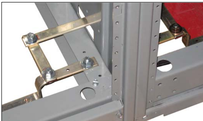
Figure 15: Series 2 Ground Bus Splice Connection
