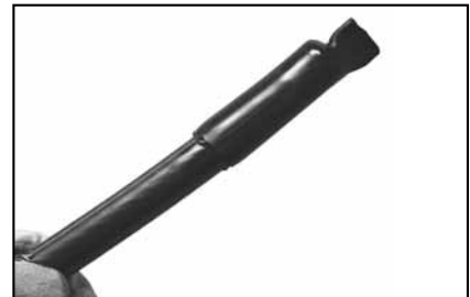
3. HSIC-FR end cap installed on cable.
