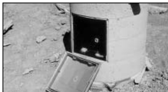
3. Pop off the J-Box lid, leaving an 8" x 8" x 4" or 12" x 12" x 4" access area, depending on the J-Box selected.
