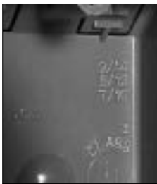
Engraved NEC Wire Fill
