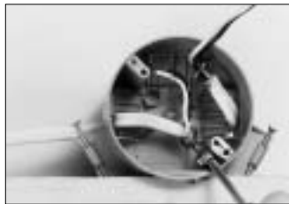
Make Grounding Connection
