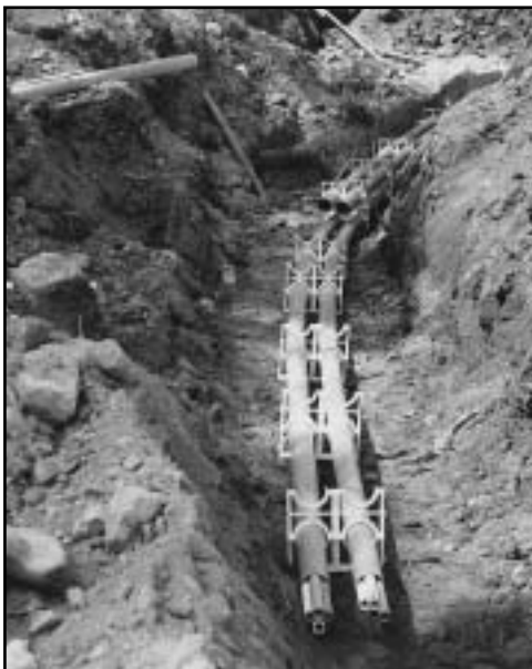
Pulled through existing conduits
