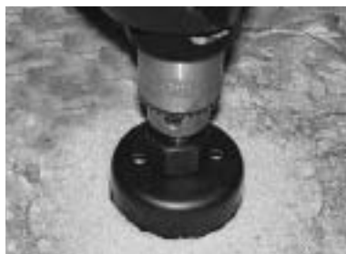
2. Drill hole in floor using hole saw.
