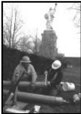
Trim spigot end before attaching pulling eye.
