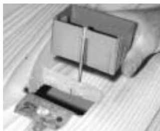
Install clip over subfloor.
