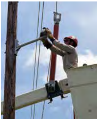
The single lifting wire holder may be rotated for alignment with the conductor.
