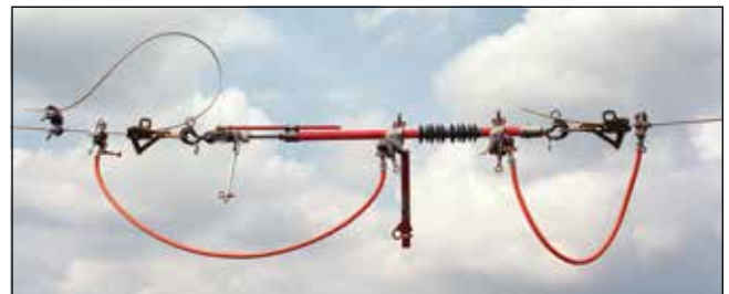
Operate disconnect switch with only a portable loadbreak tool.
