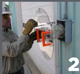
2 Closing non-conductive jaws with actuating rod
