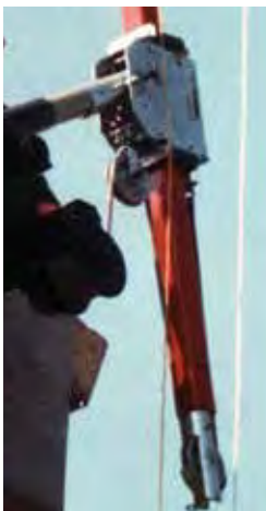
Wireholders latch easily from bucket with hookstick. 12" Epoxirod link insulates each latch-release lanyard.
