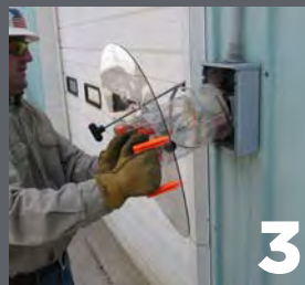
3 Removing/pulling meter
