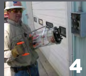
4 Meter removed from socket base
