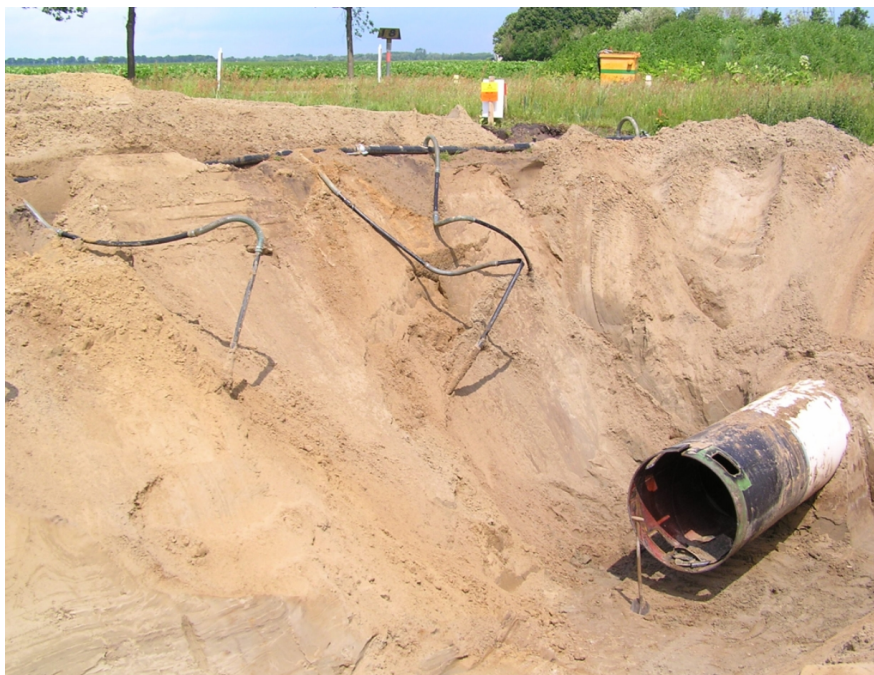
Figure 1.9: Pipeline installation in trench
