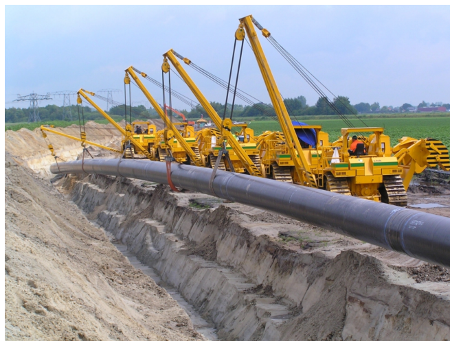
Figure 1.6: Pipeline installation in a trench
