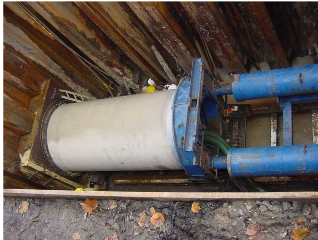
Figure 1.5: Jacking frame and micro tunneling machine in the start shaft
