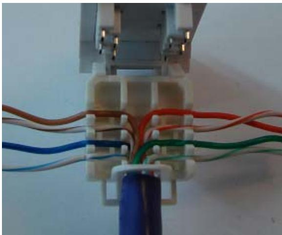
**Step 2.** Open the lid of the keystone and insert the wires through the loop at the end. Untwist and splay out the wires and sort them through the appropriate slots on the lid. Follow the color coding diagram on the side of the lid for the proper wiring standard you wish to use.
