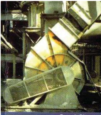
Industrial Blower: 3.3 KV, 80A, 1MW
