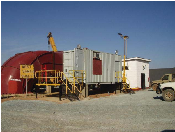
Mobile electric room for exhaust fans
