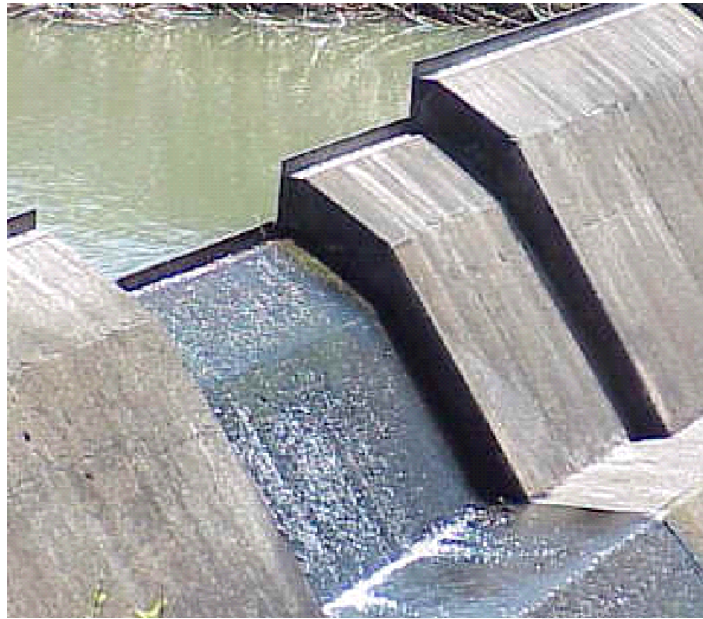
Figure 5.211: Example of a multiple-stage weir. Photo: South African Department of Water Affairs
