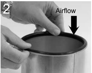
2) Carefully place the gasket along the rolled edge of the part, being careful to avoid kinks or voids. Only one gasket is needed per joint.
