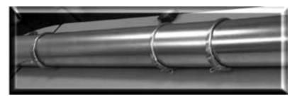
NOTE: KEEP CUT PIPE IN THE DIRECTION AS THE AIR FLOW.
