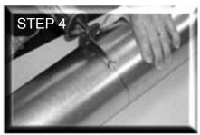
Drill access hole then cut with saw
