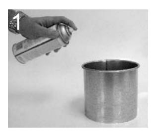
Wipe rolled edge with clean cloth. Then apply a high tack gasket adhesive per the manufacturer's instructions. High tack gasket adhesives can be purchased locally at industrial or automotive suppliers in either aerosol spray or brushable formulations.
