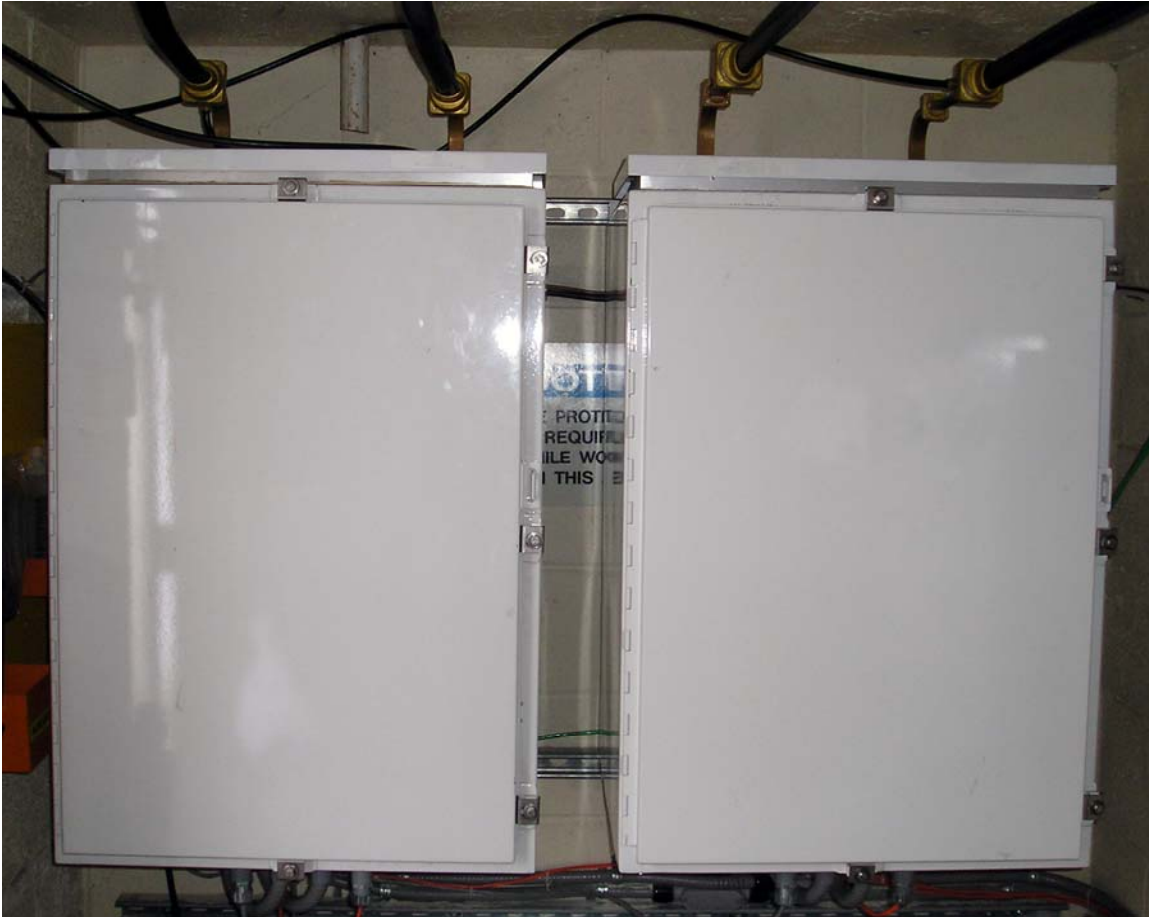
Figure 29 Example of Wall Mounting RF-11000 Repeaters. Note the use of rigid W/G bends and twists.
