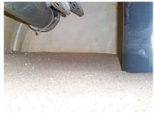
Above: Typical sand beds after draining tanks. Note the smooth, flat sand bed. There are no signs of trenching or erosion.
