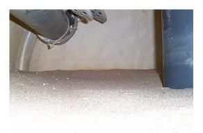
Above: Sandbed should be flat and smooth when sand is installed.
