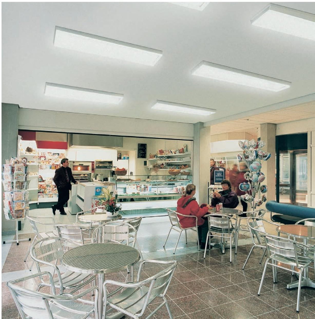
Suspended and surface-mounted luminaires
