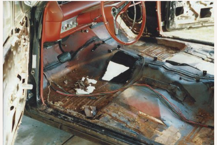
Initially, it was thought that the body mount positions and their associated braces would be primary areas of concern for corrosion; however, stripping the interior to bare metal uncovered more extensive damage to the front floorpan than previously anticipated.
