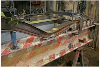
More tubing and strips of plate steel. The former was used to provide support for the latter, as the jig was carefully fabricated to match the contours of the frame. A series of clamps was used to hold everything in place while final adjustments and welds were made.
