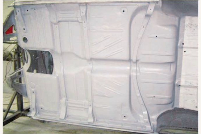
Once the numerous repairs had been completed to the underside of the Pontiac's body, its exposed metal was cleaned and given a few protective coats of self-etching primer, which was then allowed to cure before moving on to other sections.
