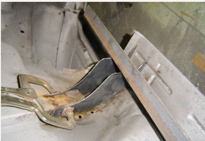
As mentioned in Part I of this restoration saga, the body mounts bore the brunt of the corrosion beyond the frame. Using what remained of the originals as a template, each had to be fabricated by different means; this one was rectified on the body.
