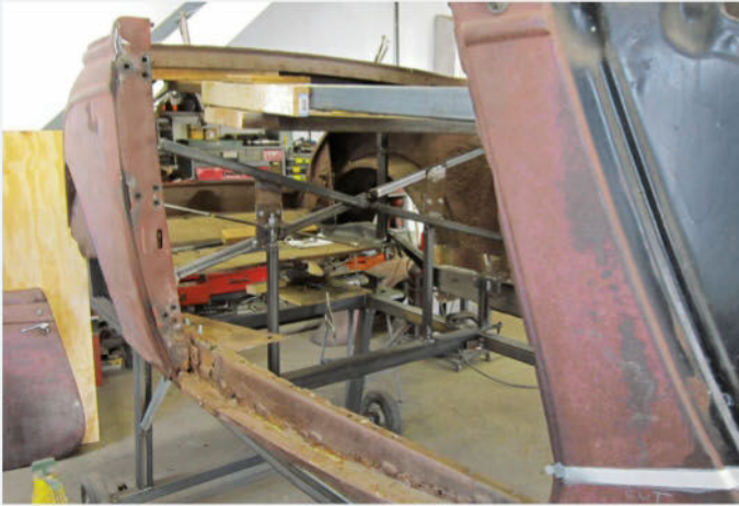
The second attempt to start the 1934 Ford Cabriolet's restoration commenced when the body was delivered without its frame. The body was secured to a purpose-built mobile jig and then thoroughly braced to prevent unwanted twisting.
