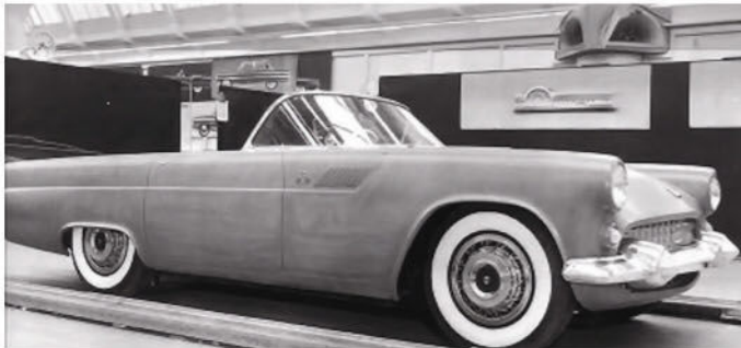
Early clay model shows original front end, with floating front bumper. Design studio staff bucked the model onto a lightweight wood frame after initial full-size drawings were approved by management. This was close to the actual production version.
