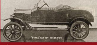
"High class English coachwork," Duple Bodies and Motors Ltd. proclaimed of the coachwork it built on Ford Model T chassis. The firm was located in North London, and its invention was that its "convertible bodies" could provide two bodies in one. The combination here was a trade van that could be converted into a two-seater in three minutes.
