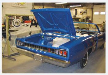
Though much of the interior, front windshield, and convertible top have yet to be fitted, at this point in the project the decklid has been installed and aligned, while several pieces of rear panel trim have been returned to the Coronet.
