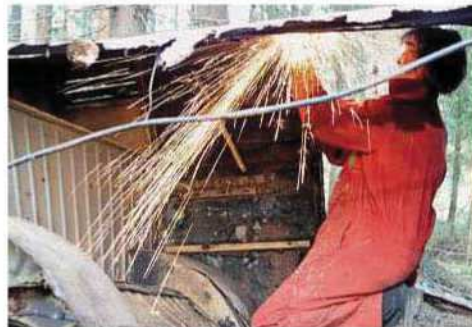
Above, left and below Bus shell was too fragile to be moved in one piece, so was cut up with an angle grinder and stacked on a trailer.
