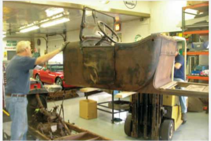
After evaluating its condition and compiling a list of missing parts, disassembly began with the removal of the turtle-deck trunk. The body was then separated from the frame and, supported by 2 x 6 boards, lifted off with the aid of a forklift.
