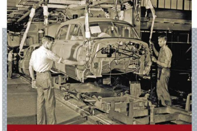
The body of this circa 1949 Cadillac is ready for transfer to a final assembly line where it will be dropped onto a waiting chassis. Note there is no structural protection ahead of the cowl, other than the sheetmetal clip that will be added down the line.
