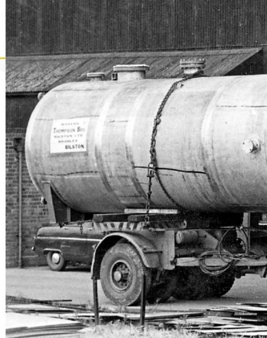
Peter standing on the step waiting to leave Thompson's of Bilston with a tank. Note the bogie just supporting end of vessel, with no trailer in between. Photo courtesy Peter Clemmet.
