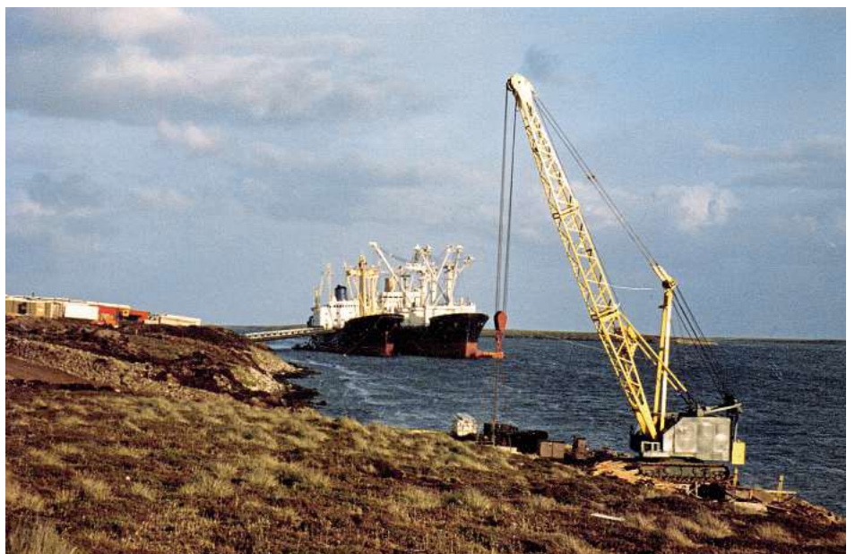
The Merchant Providence ‘jetty’ with a docked freighter at East Cove in January 1984. PHOTO JOHN BURROUGH.
