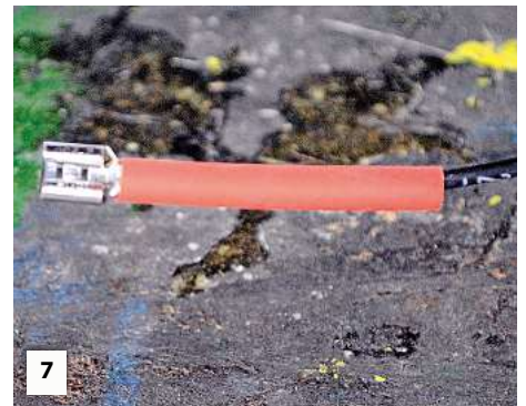
The shrink sleeving needs to be long enough to cover the soldered connection and a small amount of the wire insulation to prevent moisture being drawn into the wire by capillary action.
