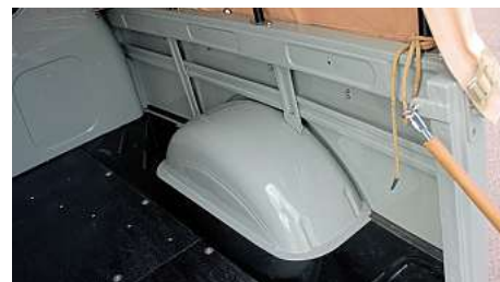
Pick-ups rot along the floor line between the 'b' post and wheel arch. Vans don't tend to suffer here.
