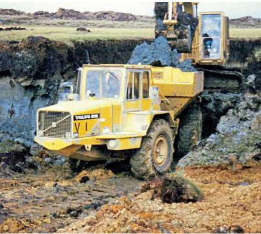
Volvo BM excavating peat. PHOTO JOHN BURROUGH.
