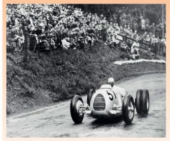
The Type C Auto Union used four rear wheels to help with traction in hillclimbs
