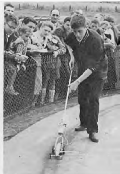
Above, Model Car Racing contributor Geoffroy de Beaufort starting his 5cc car by means of a special fork holding a battery which gives the initial ignition. Photo Geoffroy de Beaufort Collection
