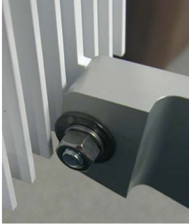
ODU bottom bracket detail
