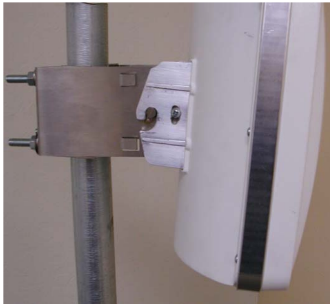
Figure 3-2: Subscriber ODU Mounting
