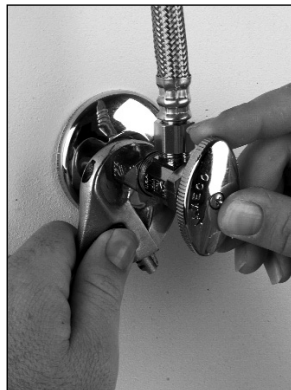
1. Turn off water supply and remove angle stops.
