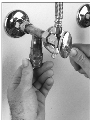
2. Install tees and attach angle stops.
