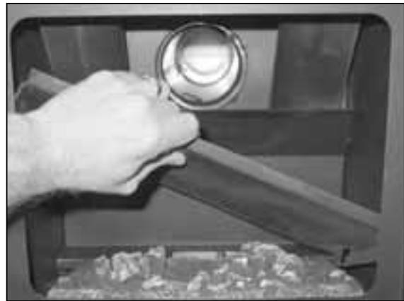
Figure 8.4 Installation of the flue restrictor requires the removal of the baffle located inside the firebox. Remove the baffle by first removing the two screws holding the baffle in place (one on each side). Lift the baffle out of the bracket along the back of the firebox, angle the baffle slightly and remove it from the firebox.
