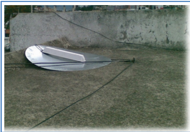
Figure 3-5: Tipped over antenna
