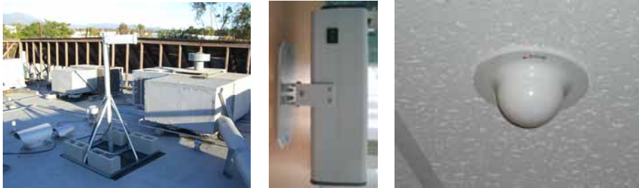
Figure 4.1 Antenna & Repeater Installation
