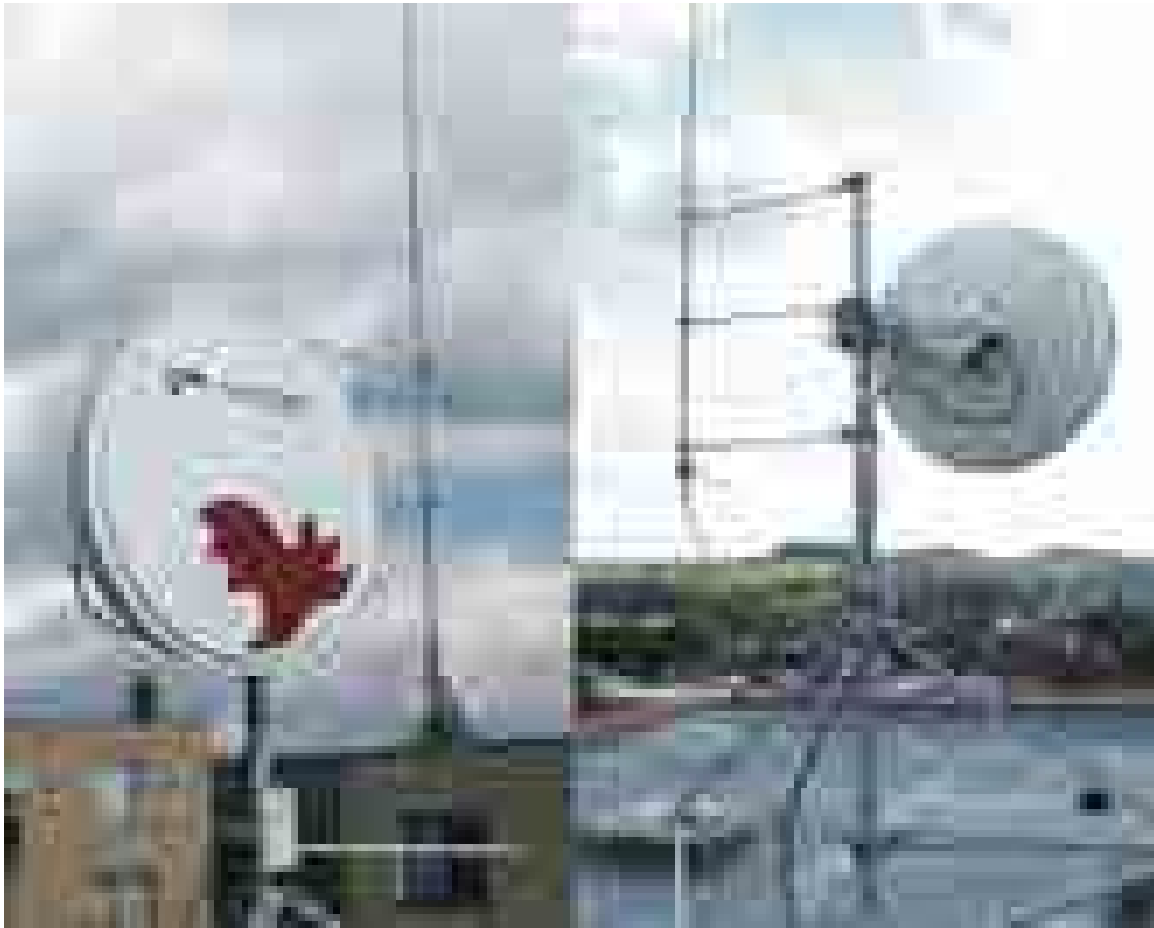
Fig. 6.36: Separated lightning conductor
