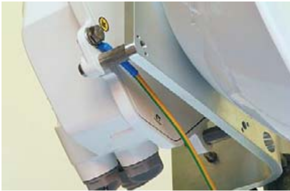
Fig. 4.9: Protective conductor at the RAY unit
