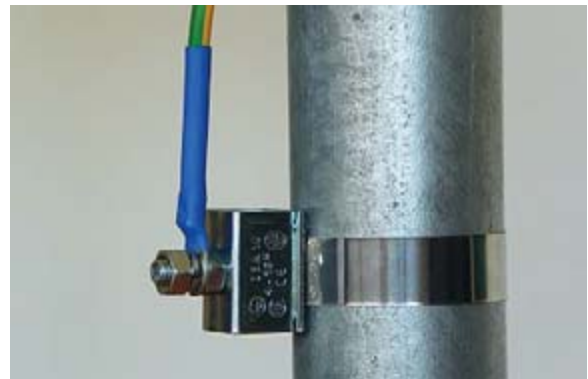
Fig. 4.10: Grounding the RAY unit
