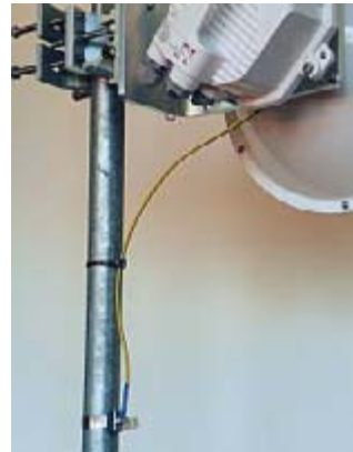
Fig. 4.10: Grounding the RAY unit
