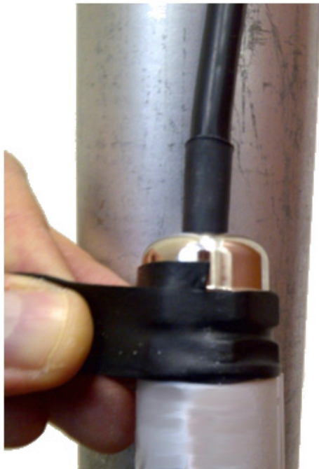
Figure 2-63: Waterproofing an external connection
