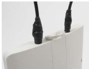
Sealing tape applied
