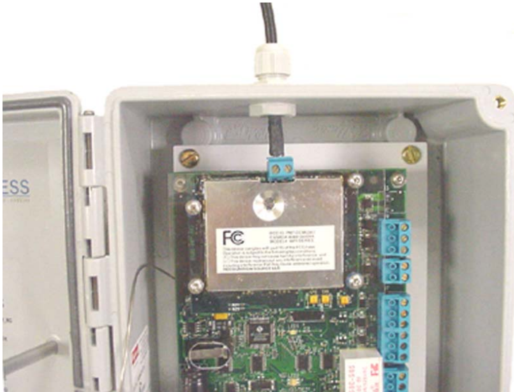
Figure 5-19 – Installing the RAM Coax in the WRI
